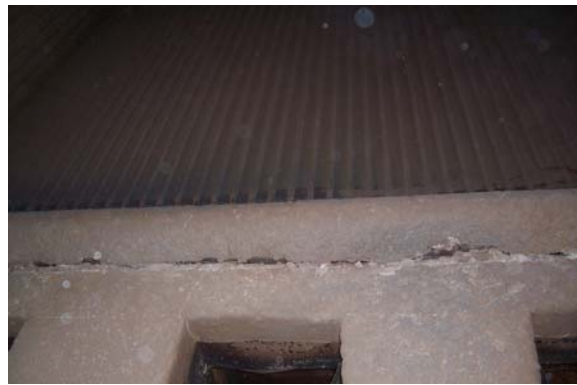
Photo 14: A clean furnace with bagasse as fuel.
