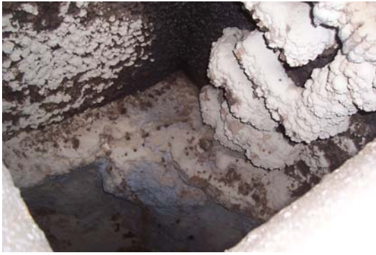
Photo 7: Ash deposition over tubes
