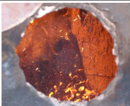
Photo 17: Poor fluidization in furnace - mal-operation
